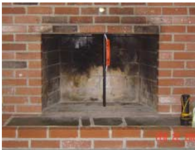
Photo #3: The Fireplace Draftstopper™ pillow is installed inside the fireplace below the damper. It is invisible unless looking up into the fireplace.
